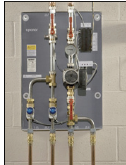
New Uponor proPANEL unit, shown without its cover
