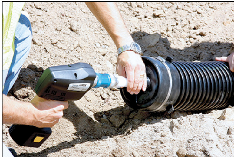
Ecoflex Potable plus works with Uponor’s durable ProPEX™ fitting system, which uses the shape memory of Uponor’s PEX-a tubing to form a fast, strong and reliable connection.
